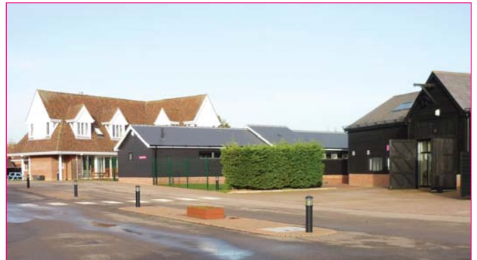
New classroom block at Eight Ash Green
